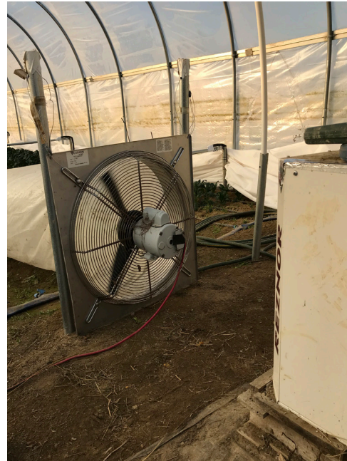
LP Gas Air Heat: Warm air from this ground level Reznor LP Gas Air Heater is funneled to the fan and pushed through the duct. The crop blanket is bunched on the far side of the tunnel in its daytime position.
